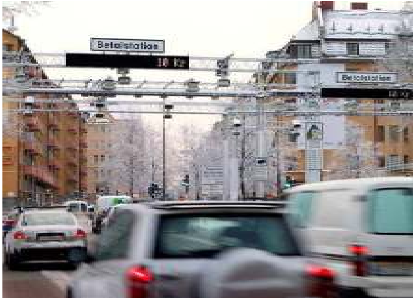
Figure 10. Congestion charge gantry in the city of Stockholm (Hugosson, 2006).
